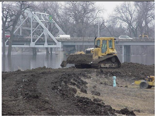
The D4 works on the dikes around the Kennedy Bridge.
