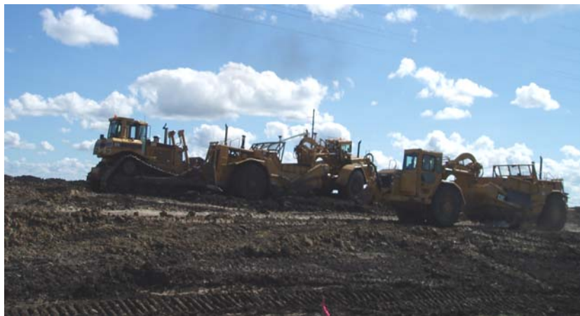
The crew at Hwy 2.
