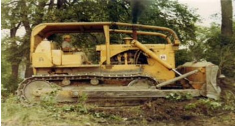
Bob Zavoral clearing a site in the early 1970's
